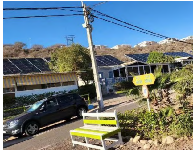
Brazil 3MW Rooftop PV Plant 5454 pcs mono half-cut 550W
